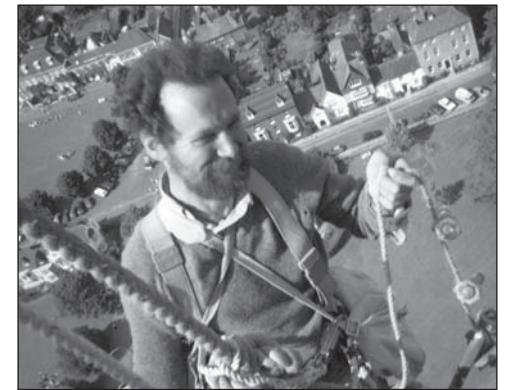
The author pictured in 1987 in a bosun's chair on the spire, during work to install the internal steel bracing
