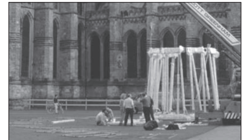
Steel brace for the middle decorative band, trial assembly on the ground
