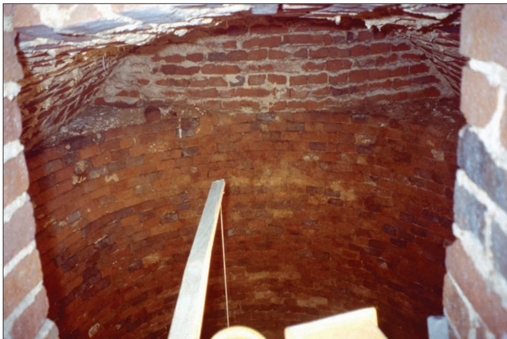
Chamber at the end of Trafalgar House drain, measuring in progress
