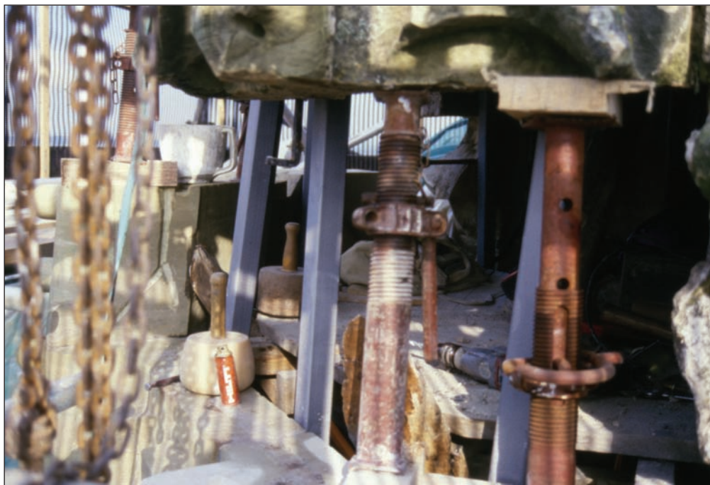
Spire upper decorated band, 180 degrees of stonework removed for replacement
