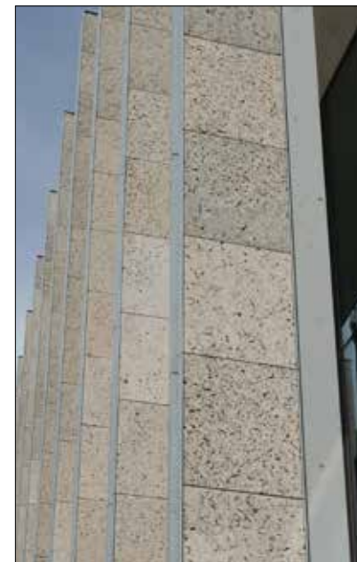
Portland Roach stone used as cladding on the extension at Bourne Hill by Stanton Williams Architects (see next page)
